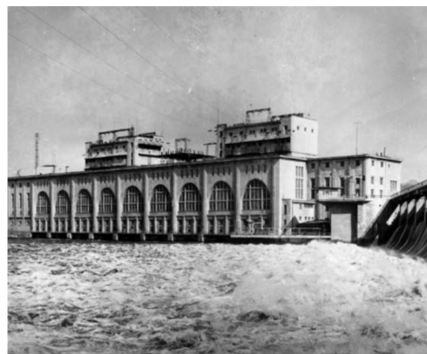
“Volkhovskaya” hydroelectric power plant
