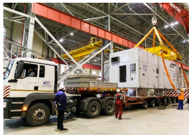
Transportation of the T16 GTU in turnkey condition
