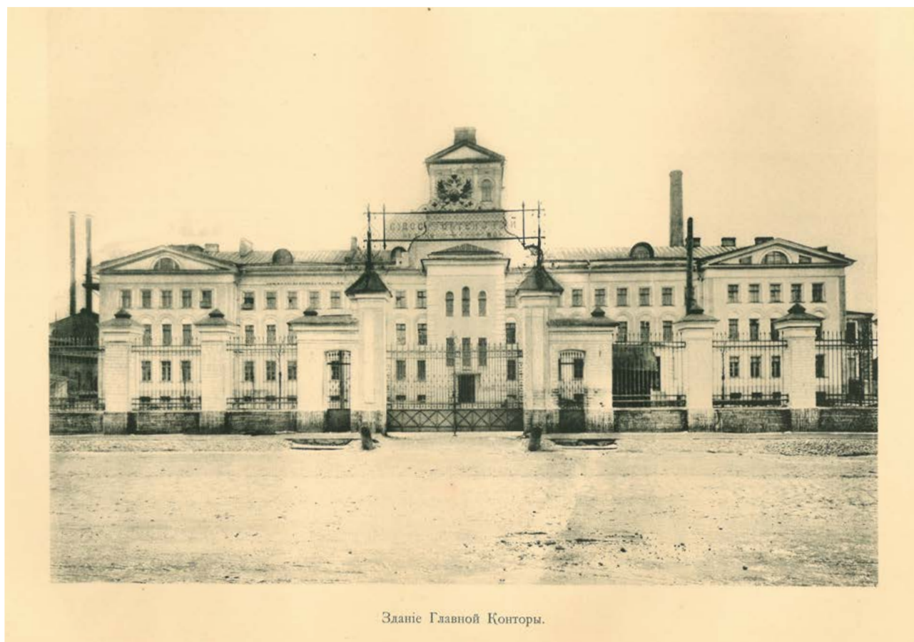
Head office building of Nevskiy Zavod, 1910
