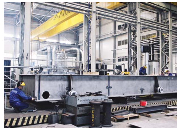
Auxiliary baseplate manufacture
